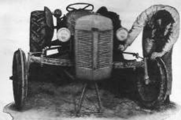
Adjusting front wheel tread width.
