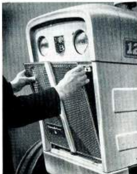
FIGURE 3/4. GRILLE REMOVAL
