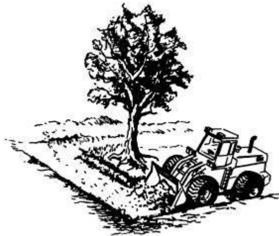
Fig. 4.41. Removing Large Trees
