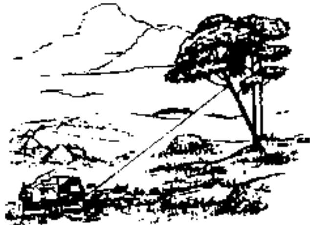
Fig. 4.39. Using Cable to Remove Trees
