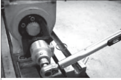
Fig. 86: Tightening the blind flange
